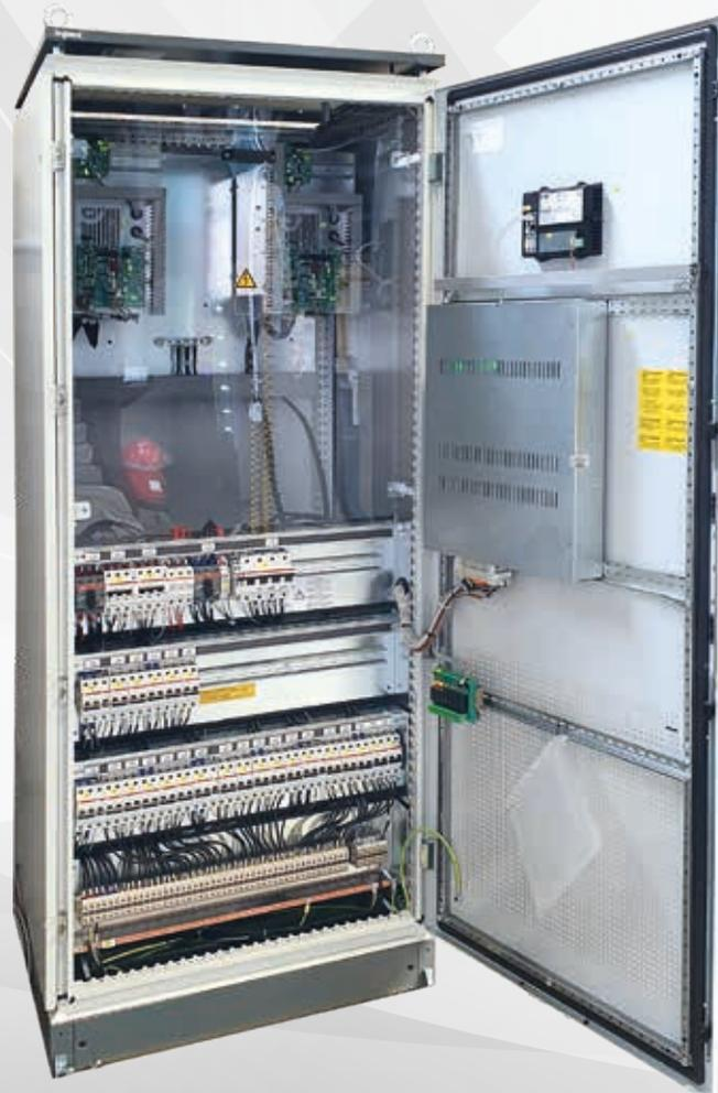
UNINTERRUPTIBLE POWER SUPPLY – UPS MTS MM/TM 3÷14KVA SERIES
